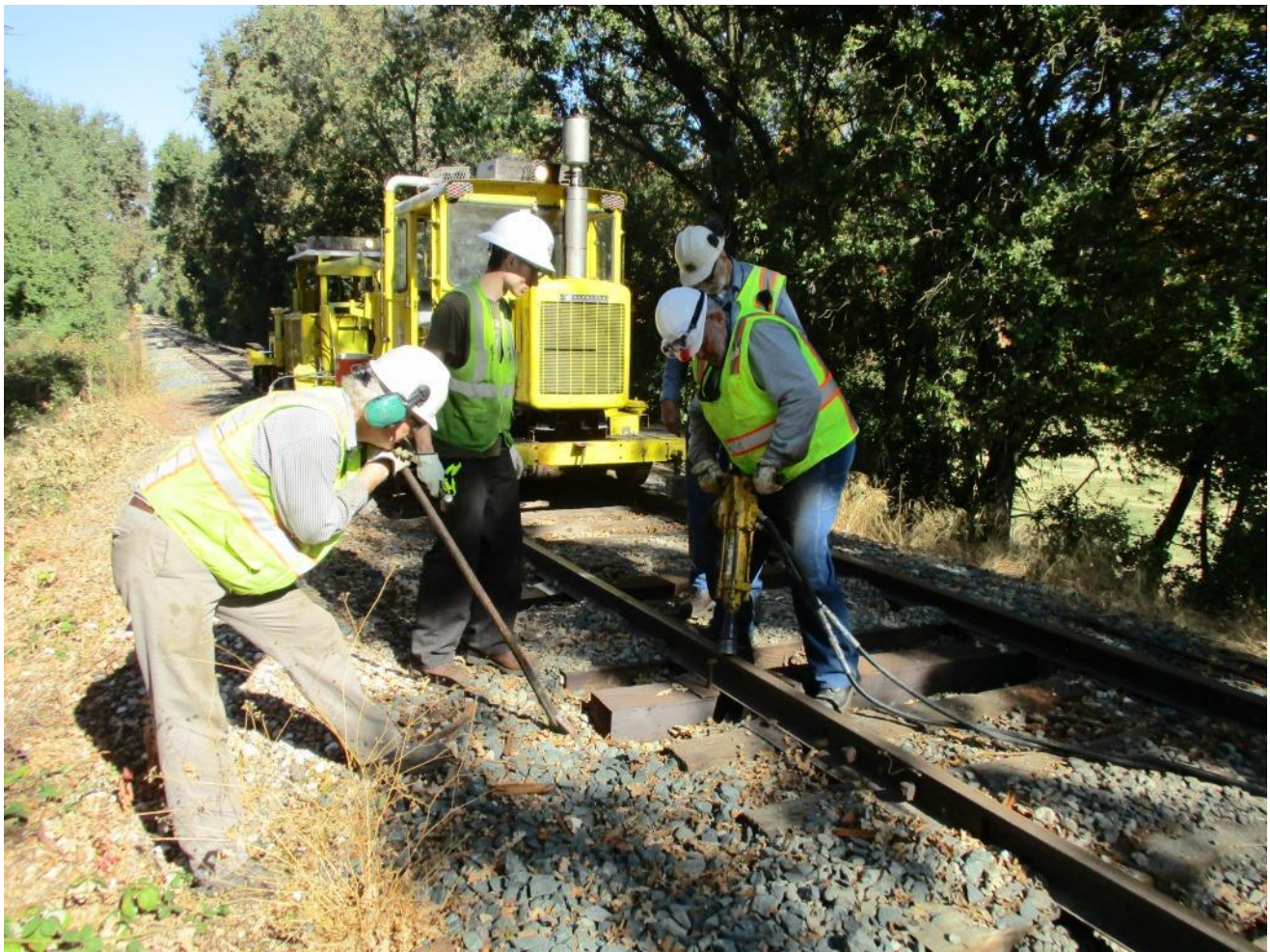
Steve N. nips-up the tie as Art drives spikes with the hydraulic spike-driver
