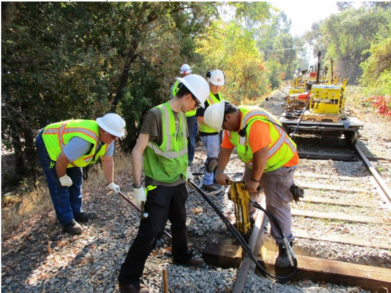
Chris nips-up the tie as Anthony drives in spikes with the hydraulic spike-driver while Paul guides the hydraulic hoses
