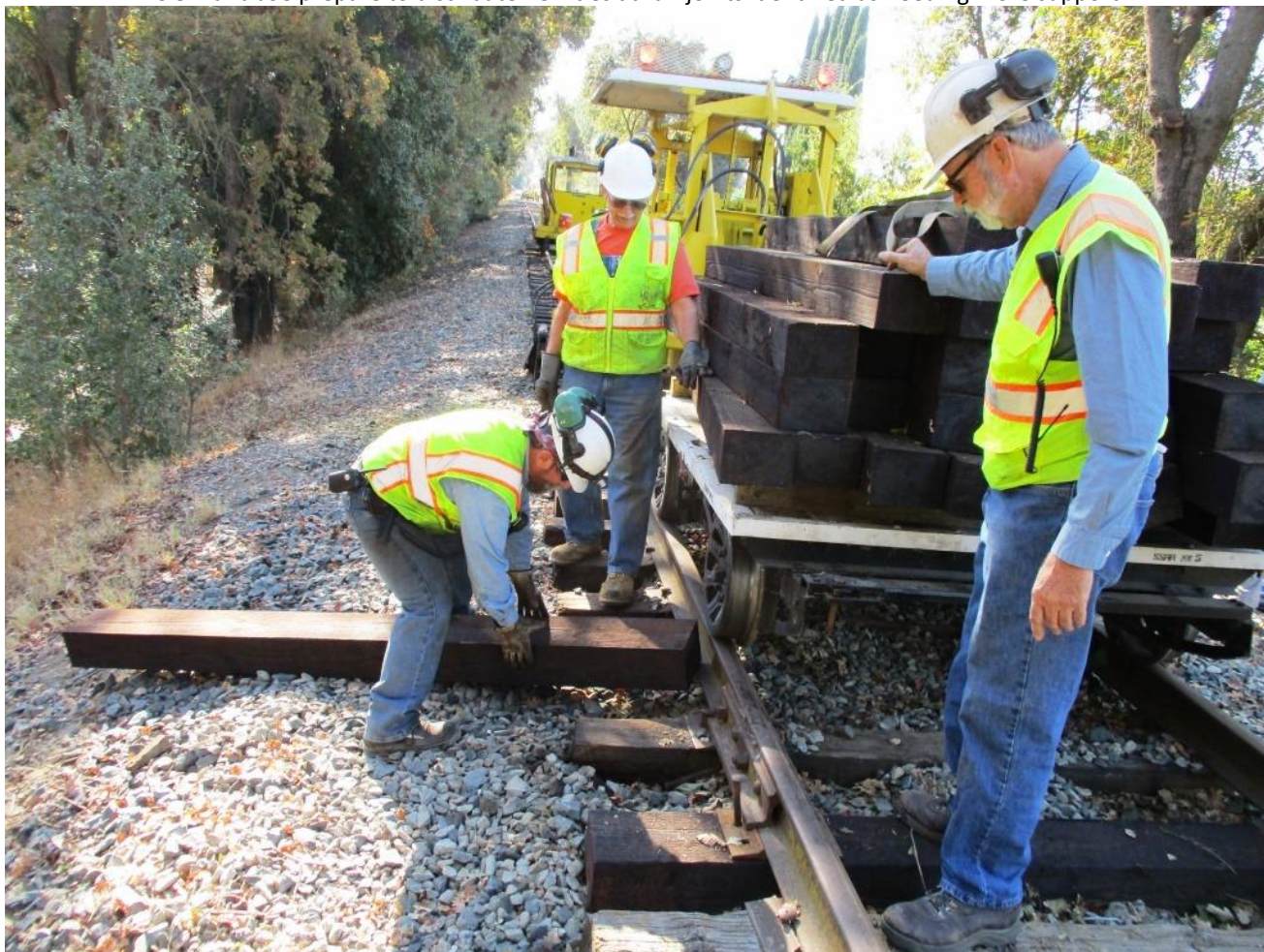
Joe lines up a tie for insertion
