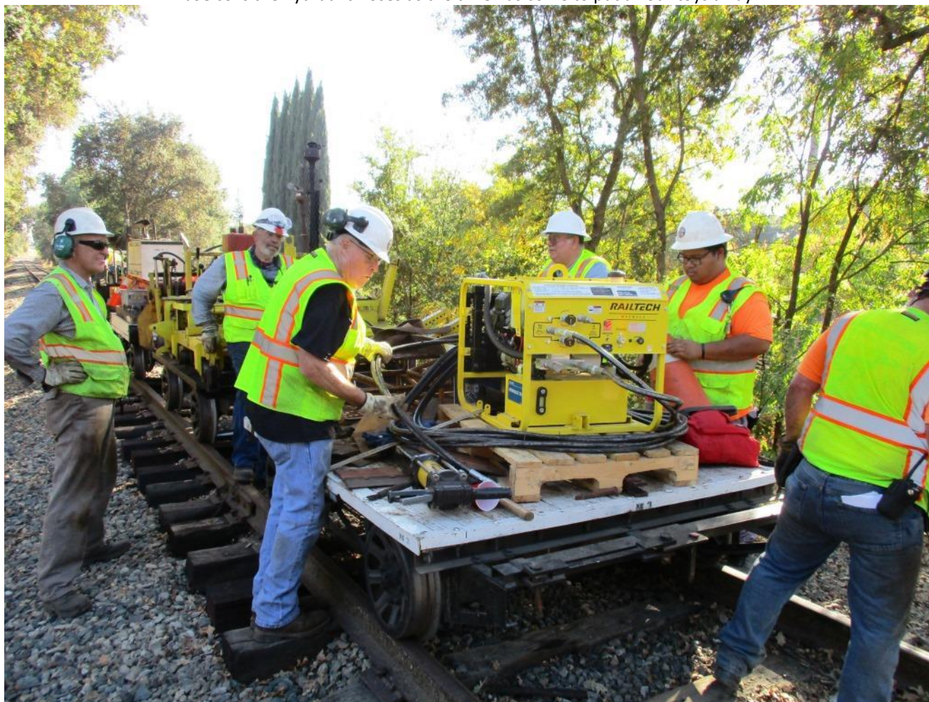
Bill and Anthony secure the hydraulic power unit to the flatcar
