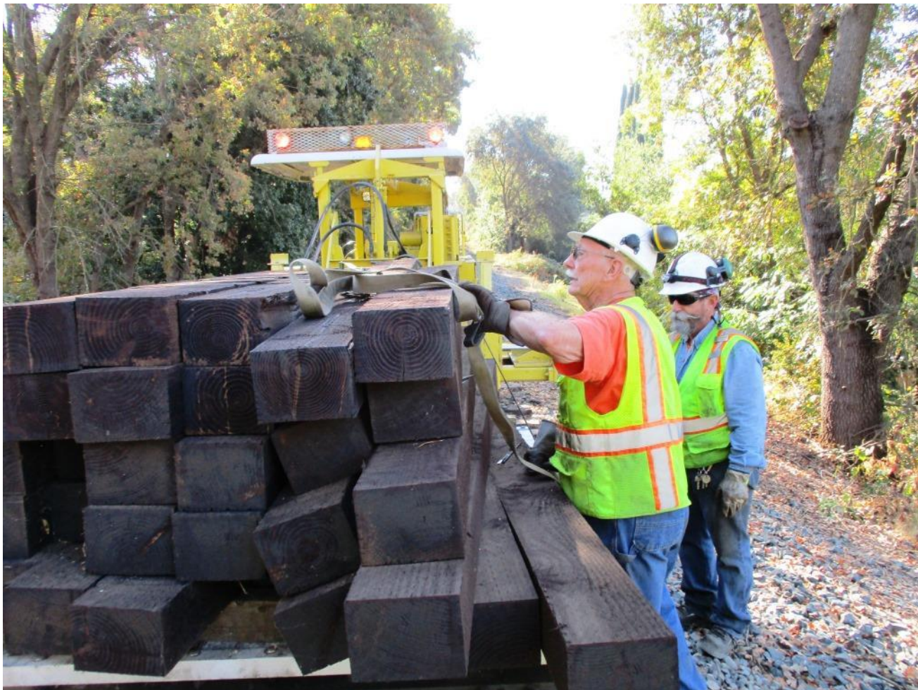
Clem and Joe prepare to distribute new ties at rail-joints identified as needing more support
