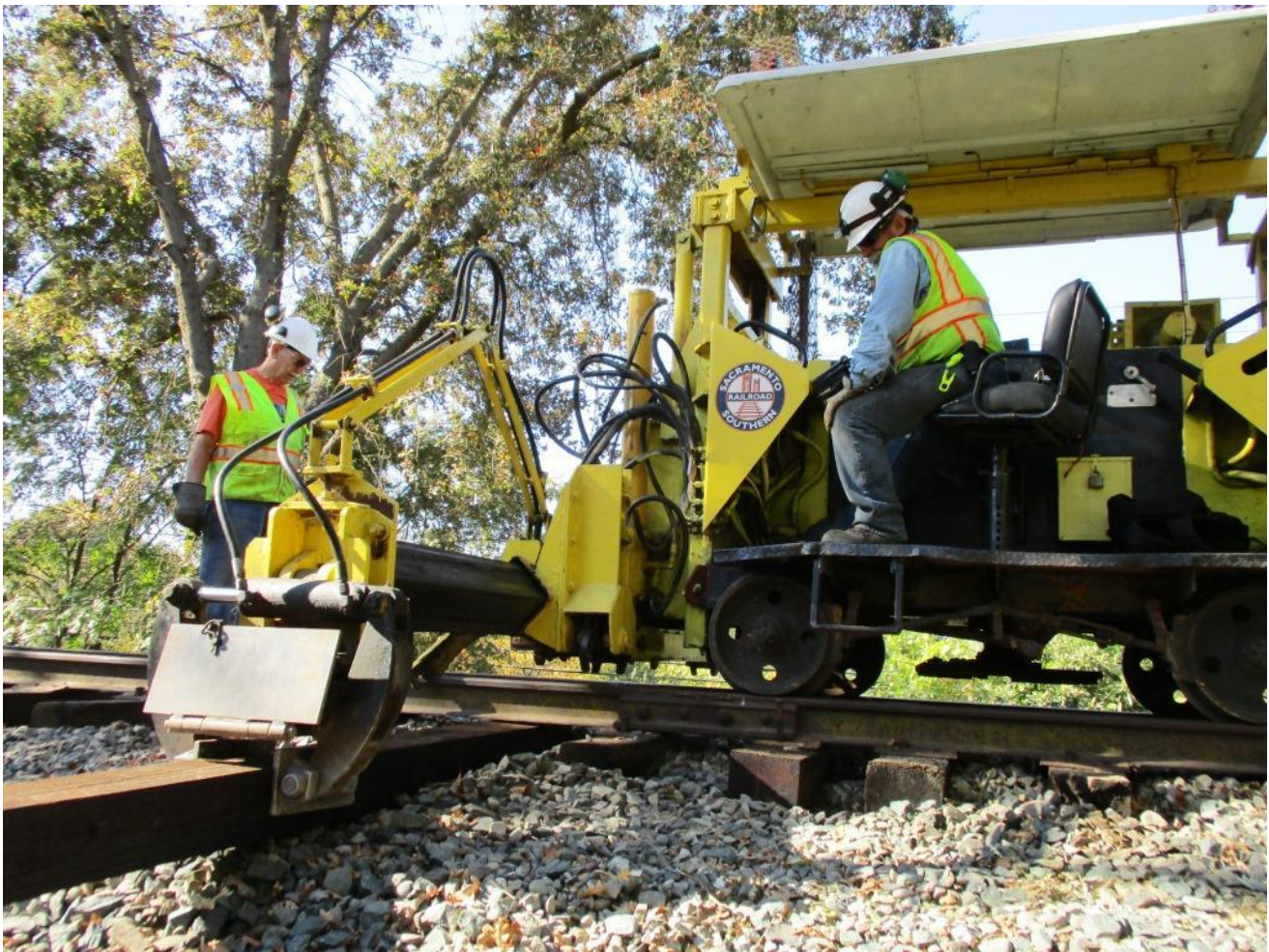
Clem keeps a close eye on the tie as Joe pulls it in with the 125 to make sure it clears the west rail
