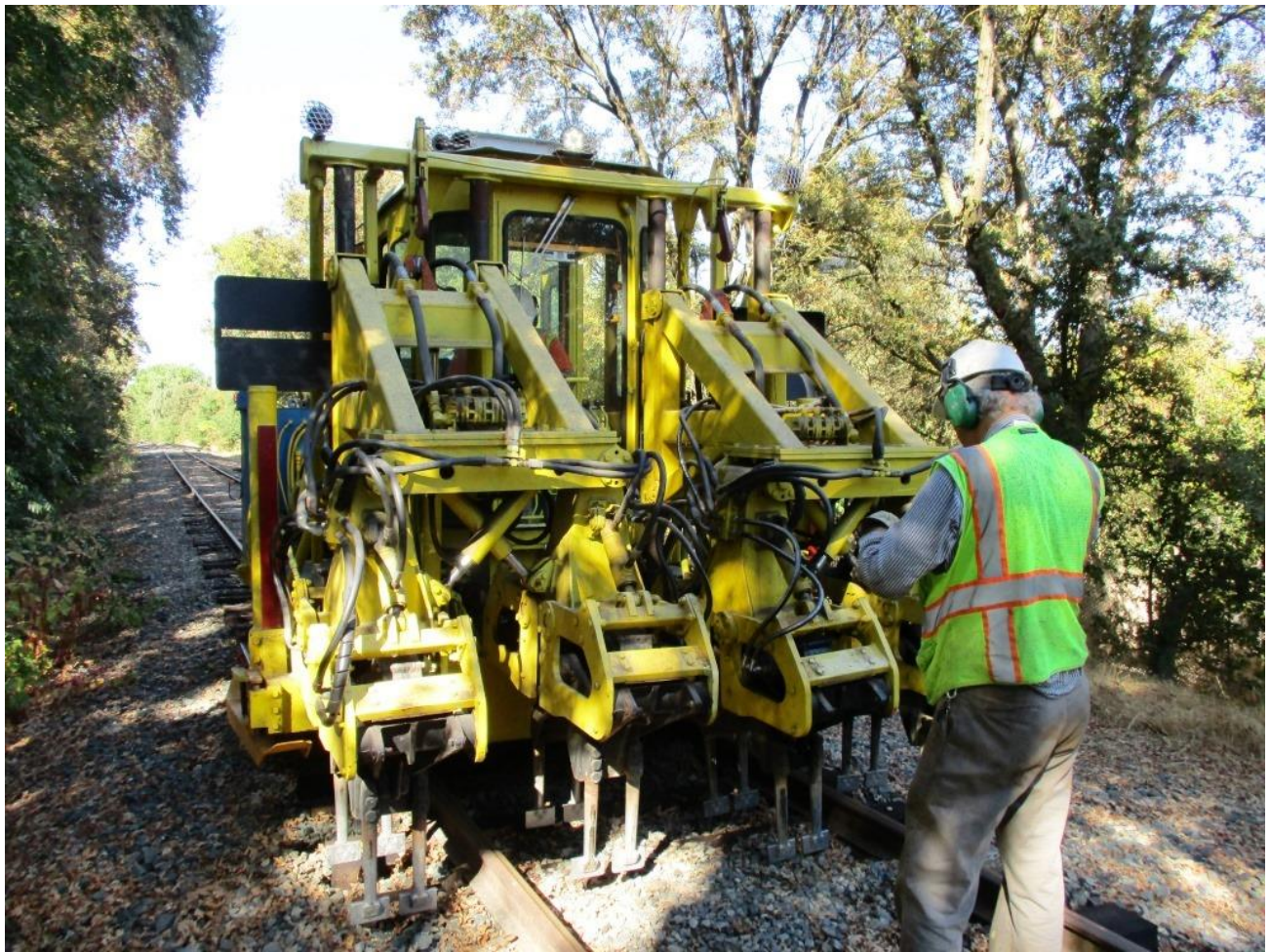
Further up the hill, Steve N. works with Harry in the tamper as they tamp the newly inserted ties
