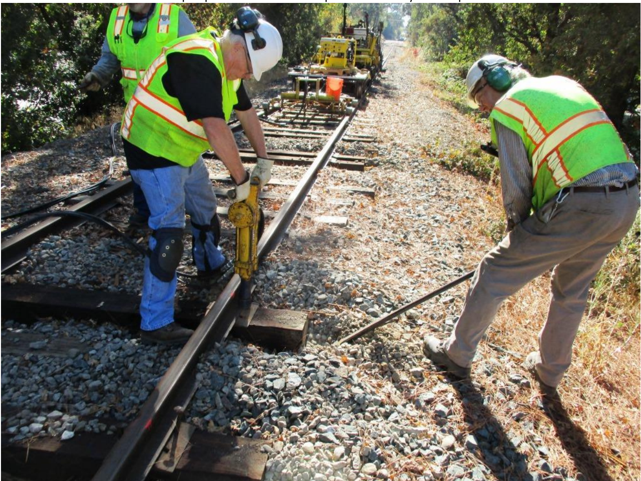
Bill takes the next shift on the hydraulic spike-driver as Steve N. nips-up the tie
